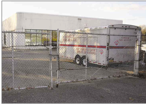
Construction on a battery storage facility in Patchogue has begun.
